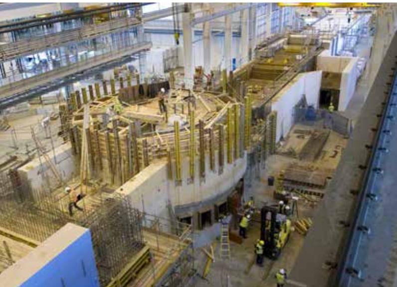
Fig. 3.21. The outer concrete layer of the TS-2 monolith (during construction)
