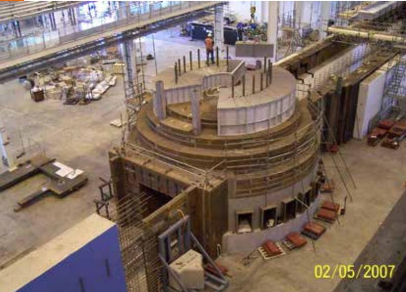
Fig. 3.20. The steel core of the TS-2 monolith (during construction).
