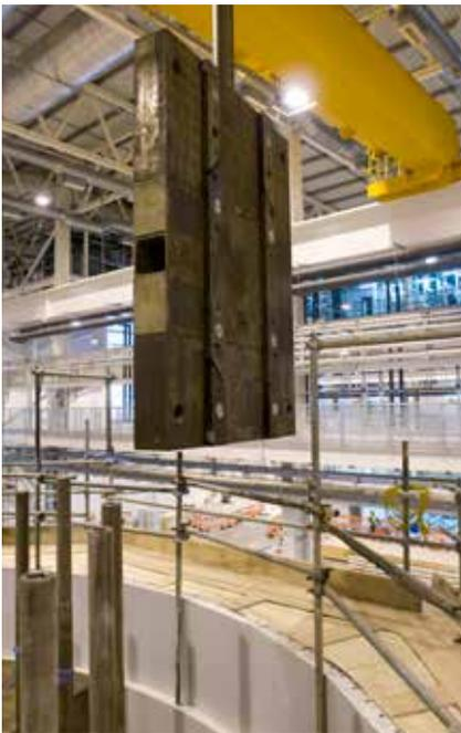
Fig. 5.1. One of the 18 beamline shutters being readied for installation into the TS-2 and then suspended from a crane during installation.
