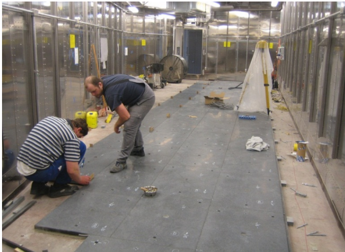
Construction of the magnetically shielded room with mu-metal
