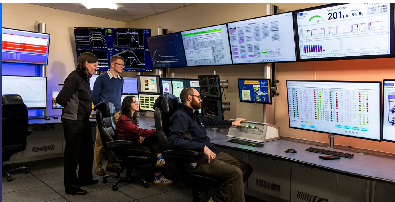
Accelerator operations being monitored in the Main Control Room.
