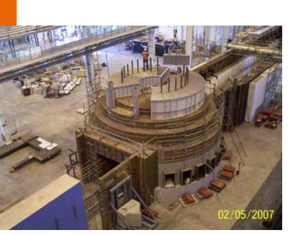
Fig. 3.20. The steel core of the TS-2 monolith (during construction).
