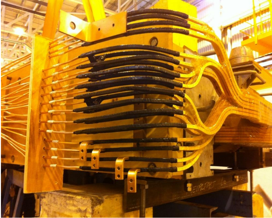
Dipole bending magnet
