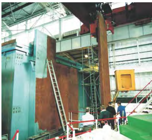
Fig. 5.10. Dismantling of the KARMEN neutrino bunker (02RC1839).
