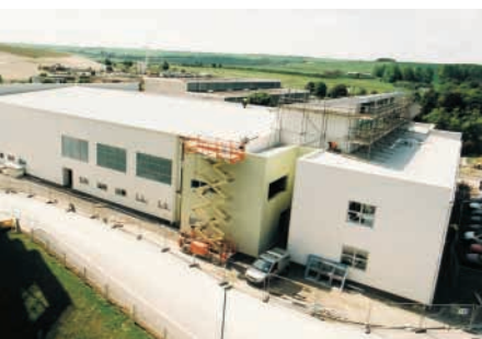
The new support services building during construction.
