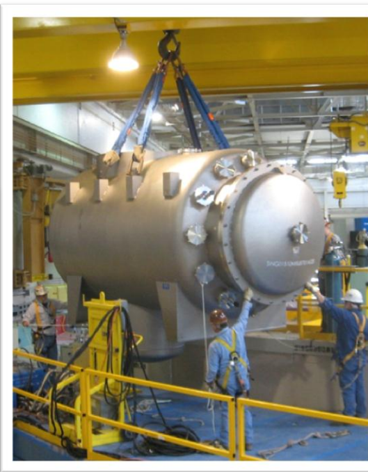
NOMAD Vessel Installation
