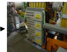
design and installation of the entire heating system :
