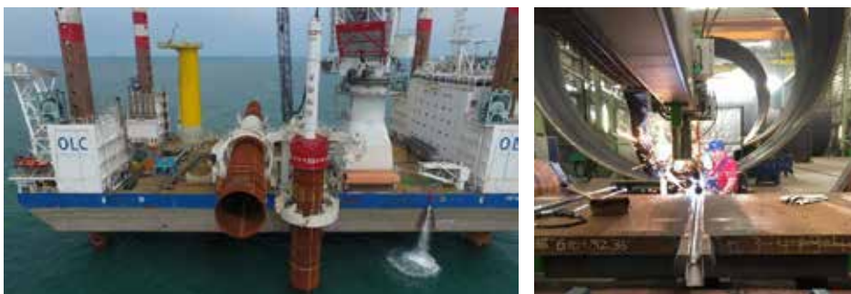
Left: The monopile, installation into the seabed. Monopile is typically 50-70 m in length and 3-10 m in diameter. Right: Monopiles are made of thick hot-rolled structural steel plates subjected to cold-rolling and bending followed by welding in the longitudinal direction to form “cans”. Image reproduced from: A. Jacob et al. Theoretical and Applied Fracture Mechanics 96 (2018) 418–427 DOI:10.1016/j.tafmec.2018.06.001
