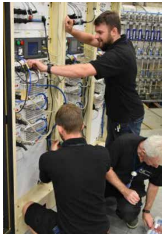
Magnet power supplies group staff Jaysen Tydeman, Michael Julian and Noel McNamee, installing a trim quad filter unit.
